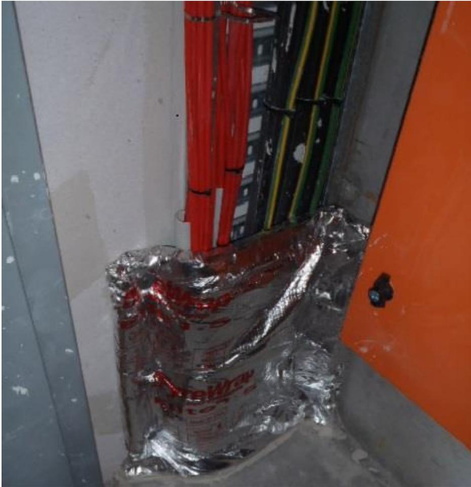
*An opening in a fire rated floor slab containing electrical services, protected with fire stopping solutions and with Fyrewrap insulation ensuring the requisite FRL of -/120/120 was maintained*
