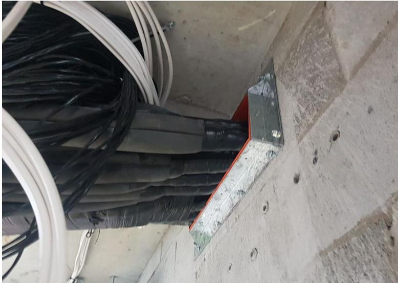
*Trafalgar FyreBOX Maxi multi-service transit protecting a glut of services passing through a fire wall. FyreBOX with these types of services have in fact been successfully fire tested and comply with NCC requirements.*
