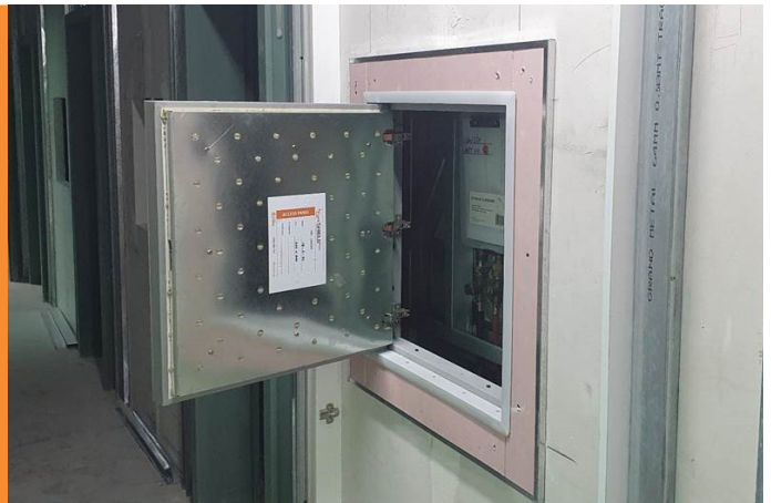
Installed FyreSHIELD Plus
