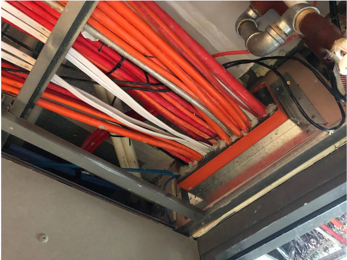
Another real life and typical application for the Trafalgar FyreBox range – again before application of FyreWRAP or TWRAP
