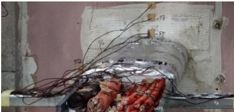
A cable tray with a large assortment of cables being fire tested; please note AS4072 Part 1 provides some acceptable and typical installations that require fire testing; again, please note the fully encapsulated Trafalgar TWRAP. It allows relatively short lengths to be provided and is thin and easy to wrap around services.
