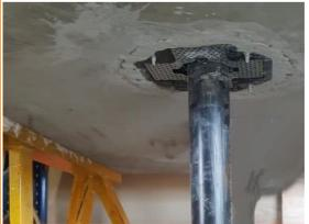
Knock the pipe down through the collar and connect the intended pipe.
