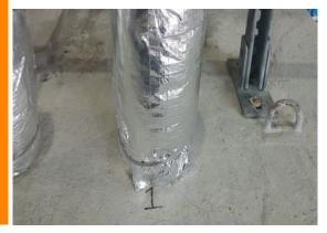
TWrap is wrapped around the service, to the approved length, secured with 4.6mm steel ties, 50mm from each end and 150mm centres in between.
