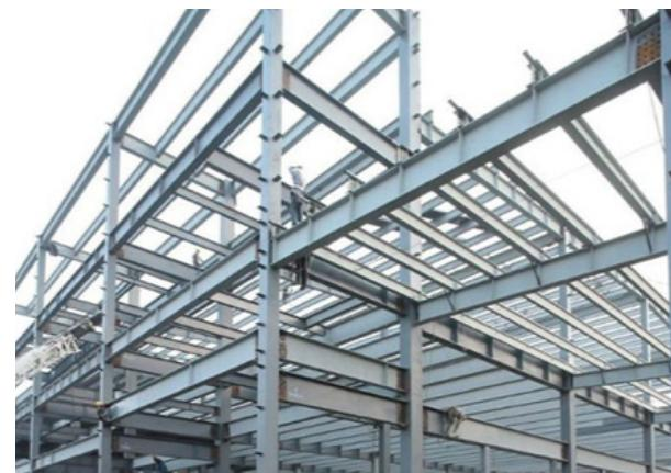
This FRL given dictates the time that the steel member is required to remain under a certain critical temperature. This critical temperature is commonly accepted to be 550°C for columns and 620°C for beams. The factors that will determine how long a steel member can remain under this critical temperature are; the thickness and quality of the fire proofing material, and dimensions of the steel member.
