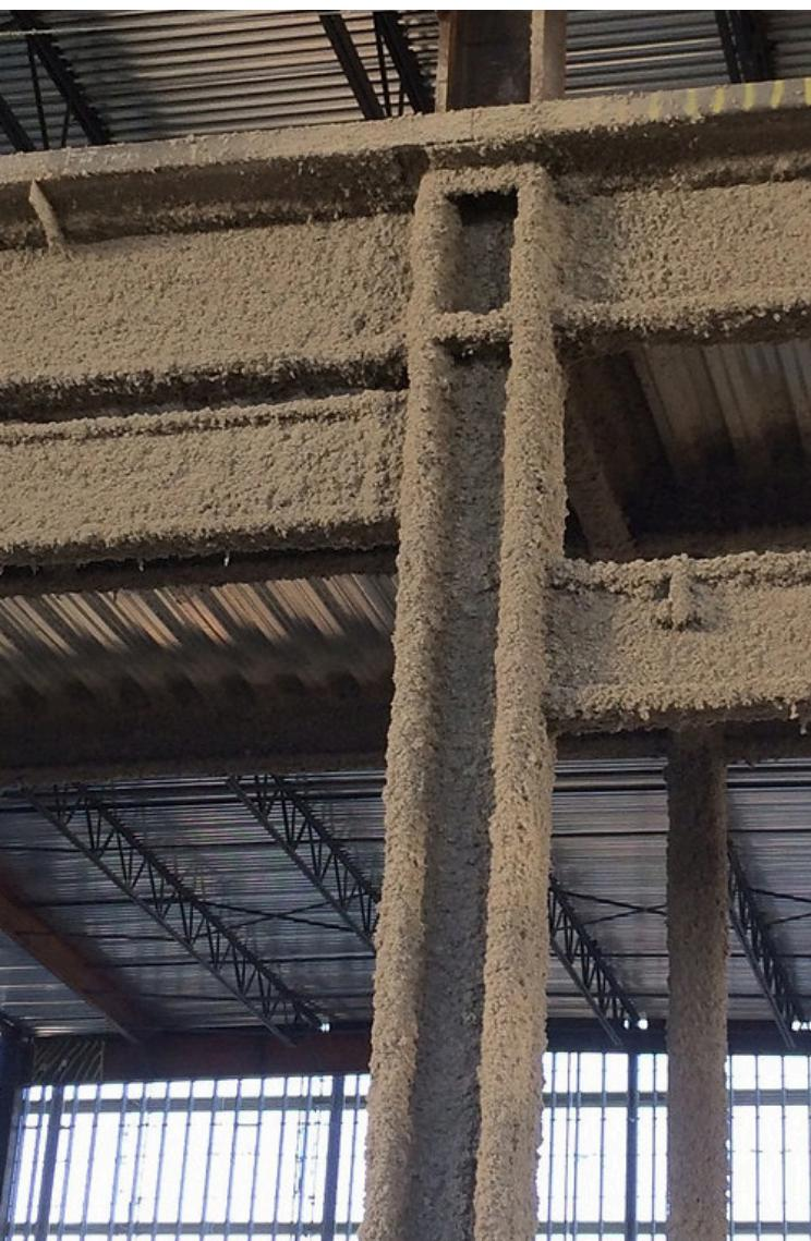
Note: Columns are calculated at 550°C critical temp, and Beams are calculated at 620°C critical temp.
