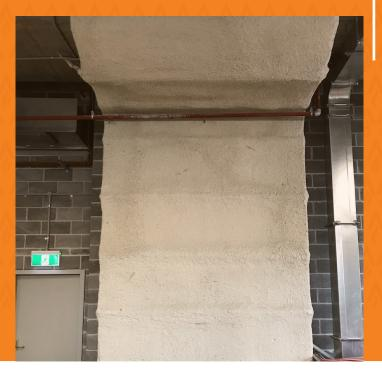
MONOKOTE® is an industry-leading fireproofing fire spray for the protection of steel ductwork which brings with it over 50 years of proven performance in the field.
