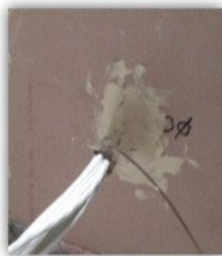
Small cable bundles don't require additional TWrap
