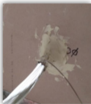
Small cable bundles don't require additional TWrap
