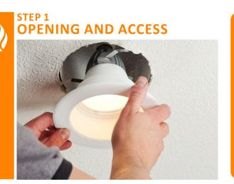
Cut and fit the downlight, speaker or other fixture to the ceiling. Do not connect the power cables yet.
