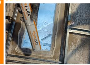
Bed the base of the DLB or top of ceiling with a gasket of FyreFLEX sealant, and place the DLB box on top of the ceiling
