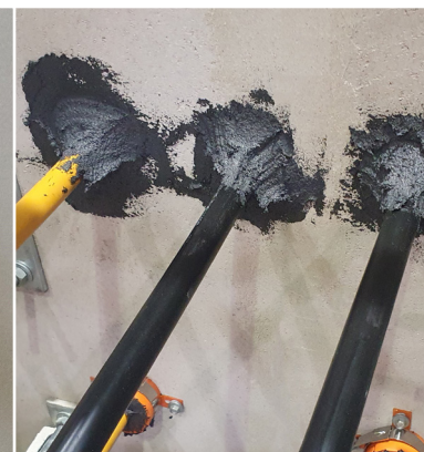
FyrePEX™ HP applied to depth of at least 60mm from top side of the wall.
