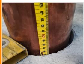
Form the correct sized hole per the approval's tables above, then the service can be run through the concrete slab.
