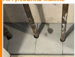
The 60mm FyreBOARD Maxilite®can be pre-cut and joined around the service. Ensure the board overlaps the slab by 100mm and fix board to the slab with M6x100mm masonry anchors. Also fix the FyreBOARD Maxilite® down to the rear steel angle with 10g x 100mm plasterboard screws at max 400mm centers.
