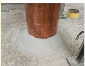
Apply FyreFLEX® Sealant to a depth of 50mm into the slab, then finish with a 30x30mm fillet on the top side. Backing rod may be used to set the correct depth.
