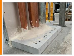
Apply FyreFLEX® Sealant to the full depth of the FyreBOARD Maxilite®, then finish with a 50x50mm fillet.
