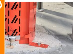
Slide the 3x fixing tabs into the preformed slots, and bend them over to hold the UniGUARD<sup>™</sup> together in shape.
