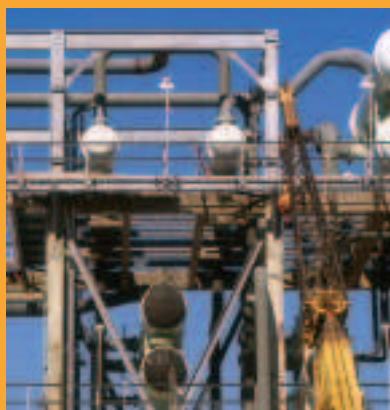
Exterior pipe racks protected with Monokote Z-146PC
