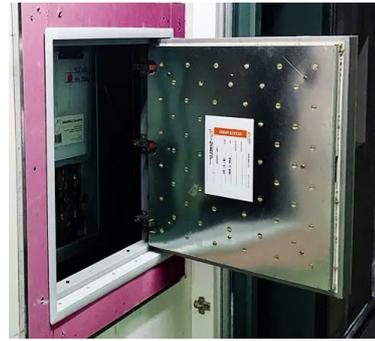
It is common on construction sites to come across service shaft penetrations that only have one sided access. This can be an issue as most fire stopping systems are required to be symmetrical and as such need access to both sides for installation. Further to this, access to both sides is often required for inspection and maintenance throughout the life of the building.
