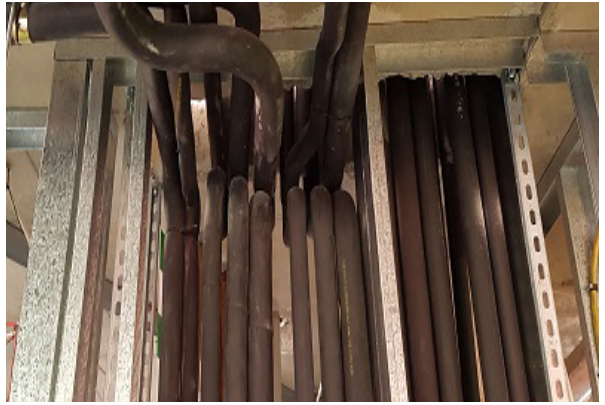
Large volumes of lagged pipes often have limited space to exit riser shaft walls, and above apartment doors. Penetrations often compromise the deflection head of the wall (below).
