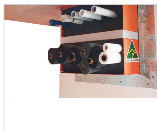
Double vertical SuperSTOPPER® installed above a doorway to allow for the provision of large amounts of services in a small space.
