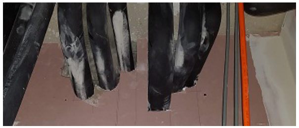
Large volumes of lagged pipes often have limited space to exit riser shaft walls, and above apartment doors. Penetrations often compromise the deflection head of the wall (below).
