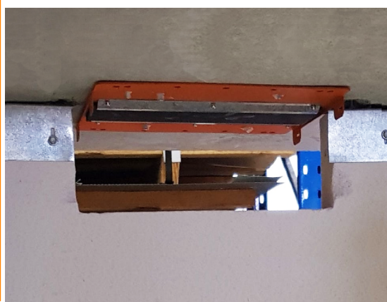
Install the Hebel® wall panel as per the supplier's instructions, ensuring the annular gaps between the SuperSTOPPER® and wall opening are within 5-20mm.
