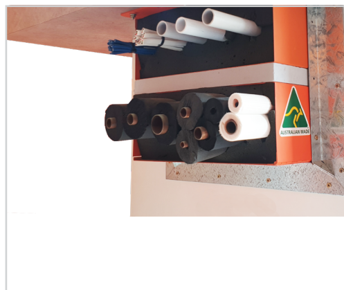
Double vertical SuperSTOPPER® installed above a doorway to allow for the provision of large amounts of services in a small space.
