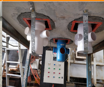
FyreCOLLAR Cast- In Floor Waste
