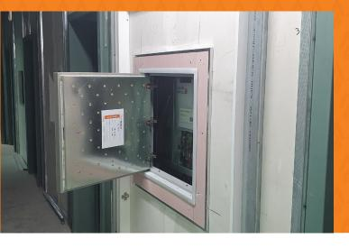
FyreSHIELD™ is a proudly Australian made access panel system which has been designed and tested to be built into partition walls and riser shafts.
