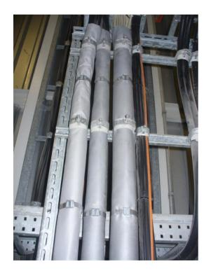
Consisting of a ready to use glass fabric, which has been treated with a specialised intumescent coating, PYRO-SAFE Cable Wraps are quick and simple to install over complex cable configurations. Cable Wraps can be removed and easily reinstated to allow the addition or removal of cables.
