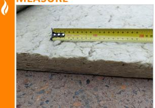
Using the table of approvals, work out what length of you MonoWRAP is needed. Measure out and mark the wrap.
