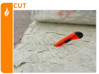
Use a stanley knife or other sharp blade to slice the MonoWRAP at the correct length.
