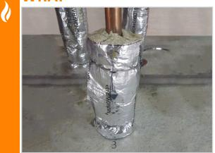
Wrap the MonoWRAP around the service penetration tightly, and strap into place with stainless steel cable ties 50mm from each end, then at 150mm centers in-between. Note that for floors, MonoWRAP is needed on the top side only.
