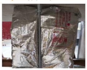
Wrap a single width of FyreWrap® around the pipe, creating a slit in the center of the wrap for the hanger to go through. Wrap the hangers the full height from pipe to concrete. Tape any open edges of wrap with foil tape.
