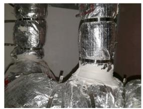
Apply FyreFLEX® Sealant to the FyreWrap® interface where the hanger meets the slab, and where the hanger meets the pipe. Nominal 20x20mm fillet should be applied. Where the pipe meets a wall, backing rod is applied in the gap (flush with the wall) and a 20x20mm fillet of FyreFLEX® sealant at the interface.
