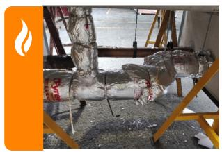
Secure the FyreWrap® with steel cable ties at 120mm centres and 50mm form each end up the threaded rod, then 200mm centres along the main pipe section.
