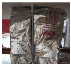
Wrap a single width of FyreWrap® around the pipe, creating a slit in the center of the wrap for the hanger to go through. Wrap the hangers the full height from pipe to concrete. Tape any open edges of wrap with foil tape.
