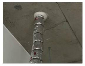
Apply FyreFLEX® Sealant to the FyreWrap® interface where the hanger meets the slab, and where the hanger meets the pipe. Nominal 20x20mm fillet should be applied.
