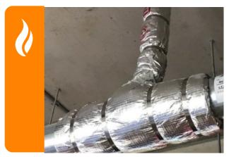
Secure the FyreWrap® with steel cable ties at 120mm centres and 50mm from each end up the threaded rod section. Also apply 4 x steel cable ties to the FyreWrap® around the pipe, 50mm from each end and either side of the support bracket (as shown above).
