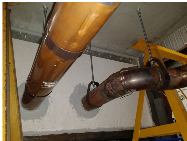
Unwrapped hydrant pipes
