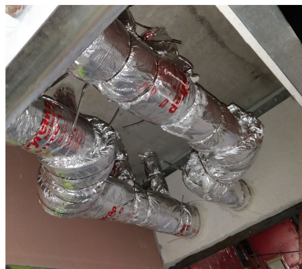
Hydrant pipes wrapped with FyreWrap within the fire compartment
