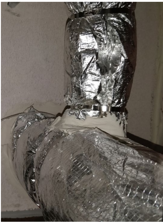
FyreWrap Critical Services Protection Wrapped around the copper pipe and steel hangers to protect the hydrant system
