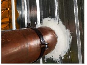
Apply FyreFLEX® Sealant to the depth specified in the approvals <u>page 12</u>, ensuring the correct size of fillet (or cone). **Sealant needs to be applied to both sides of a wall penetration.**
