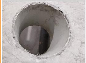
Form an opening appropriate for your service per the approvals table on page 9. Maintain 50mm between openings if multiple pipes are present. Remove any PVC formers, dust and debris.
