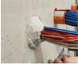
Apply FyreFLEX® Sealant to the depth specified in the approvals <u>page 16</u>, ensuring the correct size of fillet (or cone). **Sealant needs to be applied to both sides of a wall penetration.**
