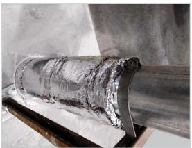
Wrap to the approved length (as per the tables above) ensuring that where the wrap meets itself, there is a 50mm overlap. Close and cut edges of the wrap with aluminum foil tape and secure wrap to service with steel cable ties. See <a href="mailto:pages24-26">pages 24-26</a> for technical drawings.
