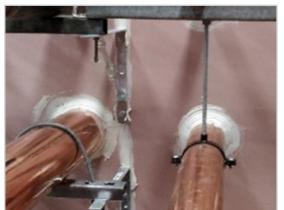
Apply FyreFLEX® Sealant to the full thickness of the plasterboard, ensuring the correct size of fillet (or cone). Sealant needs to be applied to both sides of a wall penetration.
