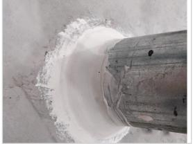
Apply FyreFLEX® Sealant to the depth specified in the approvals <u>page 11, 12 or 13</u>, ensuring the correct size of fillet (or cone).
