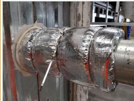
Wrap to the approved length (as per the tables on page 12) ensuring that where the wrap meets itself, there is a 50mm overlap. Close and cut edges of the wrap with aluminum foil tape and secure wrap to service with steel cable ties. See pages 24-26 for technical drawings.
