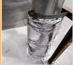
Wrap to the approved length (as per the tables on page 10) ensuring that where the wrap meets itself, there is a 50mm overlap. Close and cut edges of the wrap with aluminium foil tape and secure wrap to the service with steel cable ties. See pages 23-26 for technical drawings.
