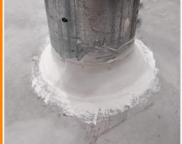
Apply FyreFLEX® sealant to the depth specified in the approvals on page 10, ensuring the correct size of fillet (or cone). Sealant needs to be applied to the top side of a floor penetration only.
