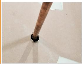
Run services through the holes formed, ensure the pipes are nominally centered in the opening. Clean the penetration of dust.
