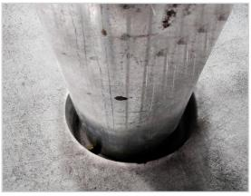
Run the services through the holes formed, ensuring the pipes are nominally centered in the opening.
