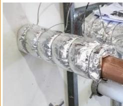
Wrap to the approved length (as per the tables on page 16) ensuring that where the wrap meets itself, there is a 50mm overlap. Close and cut edges of the wrap with aluminum foil tape and secure wrap to service with steel cable ties. See pages 24-26 for technical drawings.
