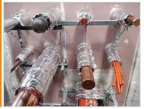
Wrap to the approved length (as per the tables on page 14-15) ensuring that where the wrap meets itself, there is a 50mm overlap. Close and cut edges of the wrap with aluminum foil tape and secure wrap to service with steel cable ties. See page 24-26 for technical drawings.
