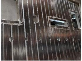
Form an opening appropriate for your service per the approvals table on <u>page 12</u>. Maintain 50mm between openings if multiple pipes are present. Clean penetration of dust.
