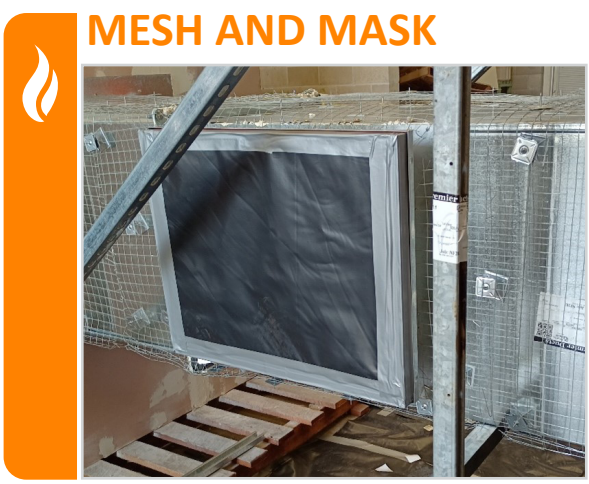
Butt the mesh to the frame of the FDAP and protect the door of the FDAP with duct tape.
