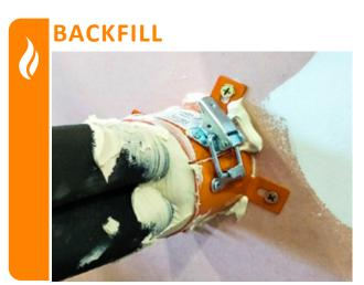
Where annular gaps exist between the services and the collar, back-fill these FyreFLEX® Sealant to the full depth of the collar.
