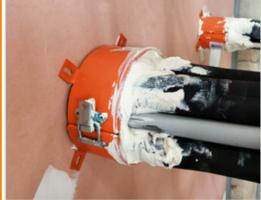
Fit the FyreCOLLAR Premium Retrofit Collar, undo the latch to open the collar, secure it around the service/s, and re-secure the latch.
