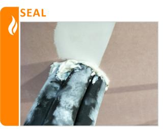
Fill the annular gap between the service and wall with FyreFLEX® Sealant for a depth of 10mm, on both sides of a wall or top and bottom of a floor.
