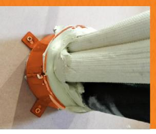
Trafalgar Fire is proud to present our newly developed Mixed Service Collar approvals for HVAC&R penetrations with our FyreCOLLAR Mixed Services. Treat multiple sets of pair coil plus their cables, insulated pipes and drain lines all through one penetration, making HVAC&R penetrations fast, clean and easy.
