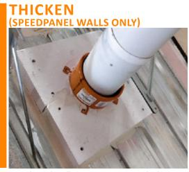
Speedpanel walls require a 60mm thick piece of FyreBOARD Maxilite® to be screw fixed onto one side of the penetration, before attaching the collar. See table below for screw fixings. Seal all gaps and perimeter with FyreFLEX® Sealant.
