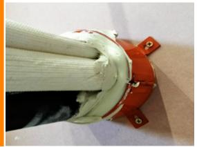
Use appropriate fixings as per page 8 to secure the collar to the wall/floor using all of the available the fixing tabs.
