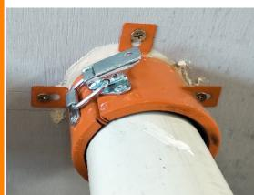
Use appropriate fixings as per page 13 to secure the collar to the wall/floor using all of the available the fixing tabs.
