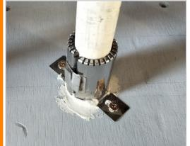
For the FyreCOLLAR Conduit, separate the two halves, fit them on either side of the service before sliding the halves back together.
