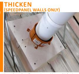
Speedpanel walls require a 60mm thick piece of FyreBOARD Maxilite® to be screw fixed onto one side of the penetration, before attaching the collar. See table below for screw fixings. Seal all gaps and perimeter with FyreFLEX® Sealant.
