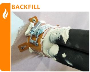
Where annular gaps exist between the services and the collar, back-fill these FyreFLEX® Sealant to the full depth of the collar.
