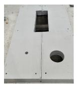
Using a hand saw, jig saw or reciprocating saw, cut the Maxilite board to the required size. It can be installed in various sections around existing services. Leave an annular gap around each service (refer to FRL tables above for maximum annular gaps).
