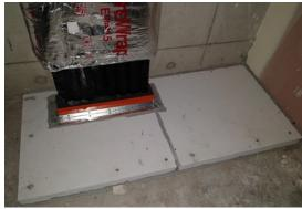
Seal any butt joints with FyreFLEX sealant, and apply FyreFLEX sealant to the perimeter of the board with a 10x10mm fillet.
