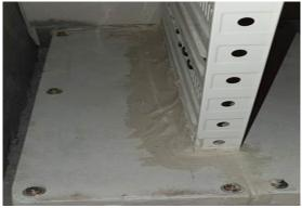
Fix the Maxilite to the wall or floor. These are to be installed 50mm from the edges of the Maxilite board and located at 400mm centers for concrete/masonry walls, or 200mm centers for other walls.
