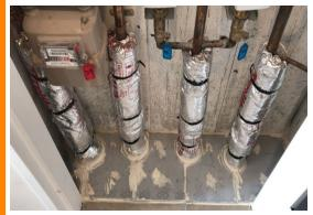
Where required, wrap the services with TWrap with a 50mm overlap, and strap in place with 4.6mm steel cable ties 50mm from each end, and 150mm centers in-between.
