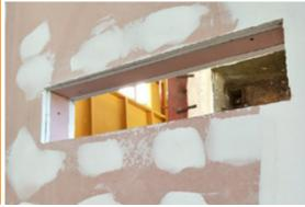
For plasterboard walls, the opening (or aperture) is required to be lined with stud framing and strips of plasterboard inside the opening.
