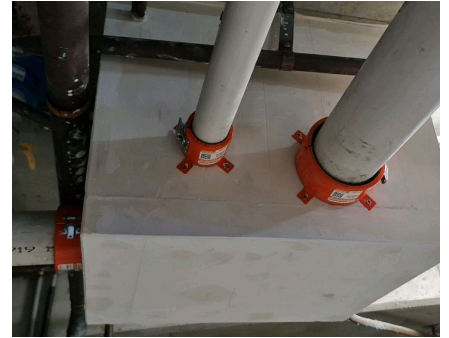
The installation process of building a compliant bulkhead with fire-rated boards can be quite tedious and expensive
