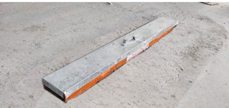
Image shows SuperSTOPPER® Cast-In in freshly poured concrete slab ready for the lid to be removed and services run.
