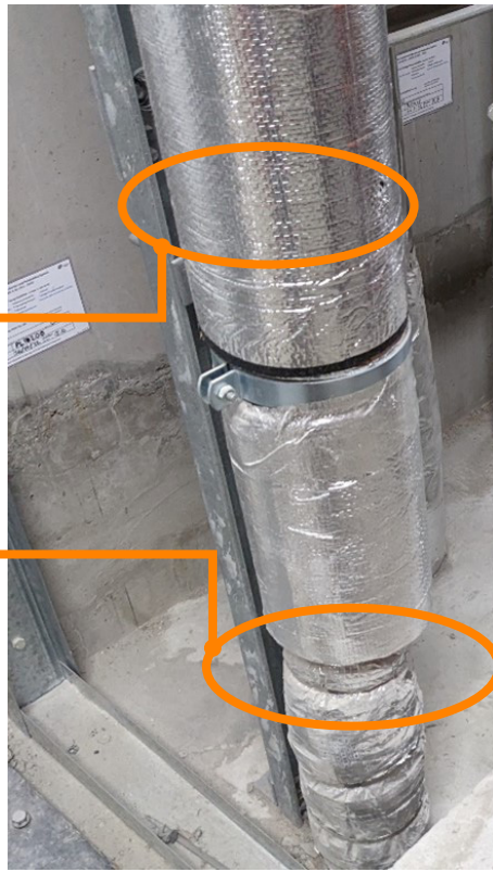
Traditional fire stop wrap with poor vapour seal
