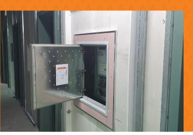
FyreSHIELD<sup>™</sup> is a proudly Australian made access panel system which has been designed and tested to be built into partition walls and riser shafts.
