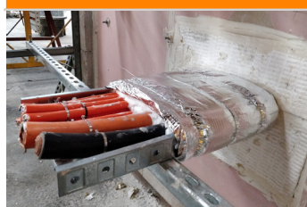
FyreBATT in plasterboard wall
